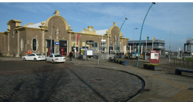
Stationsplein Station Vlissingen, 2013
