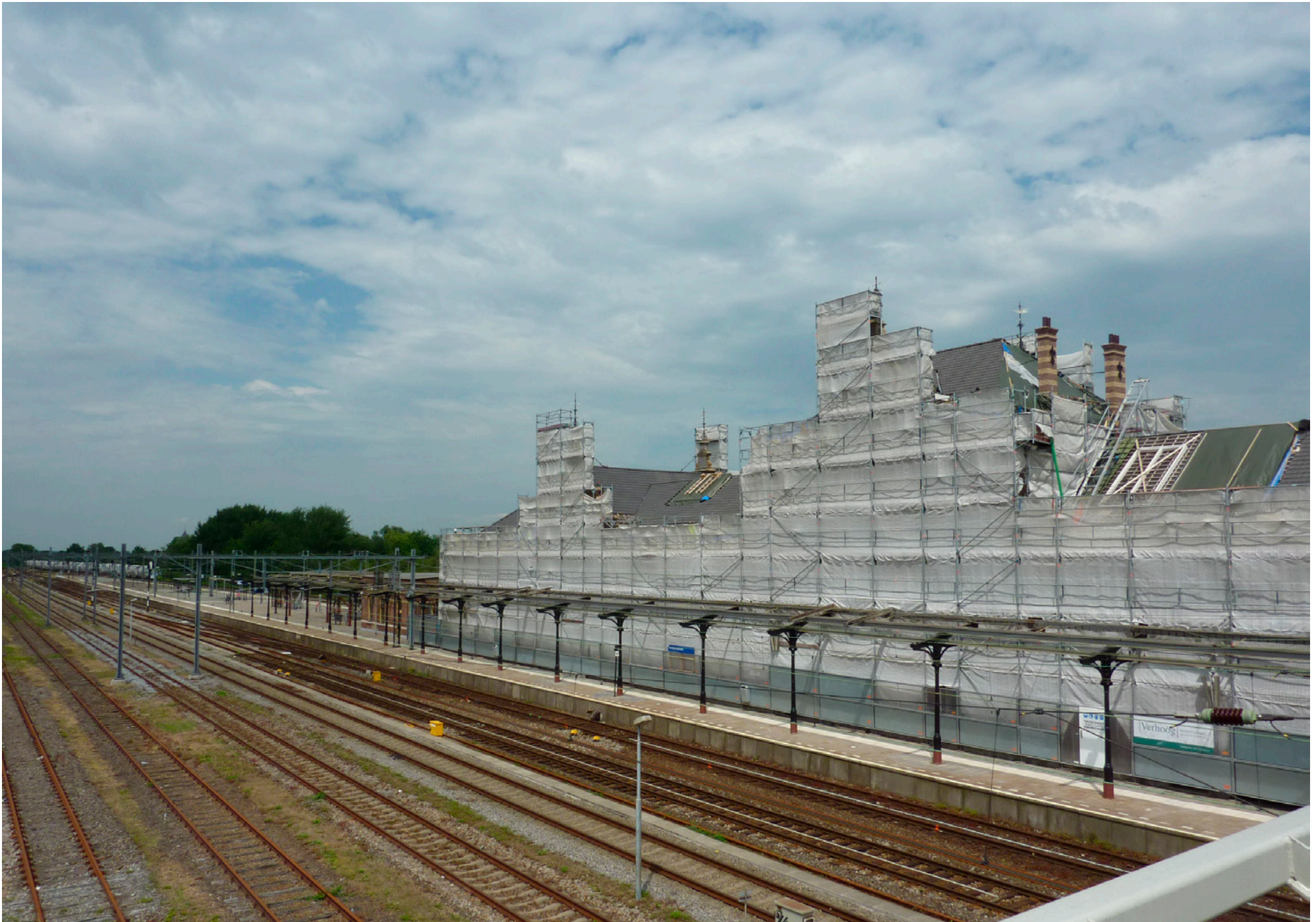
Station Geldermalsen in restauratie.
